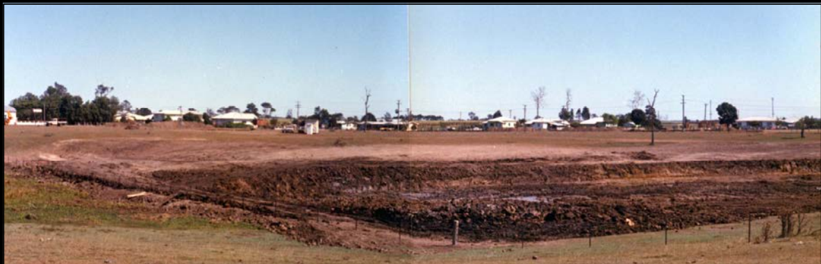
bun02808 Excavating Lake 2 at the Botanical Gardens June 1984
