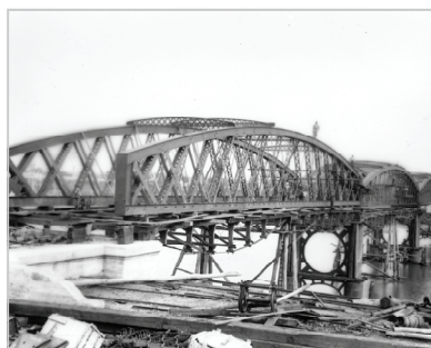
ca1900 - The bridge nears completion. bun01086
