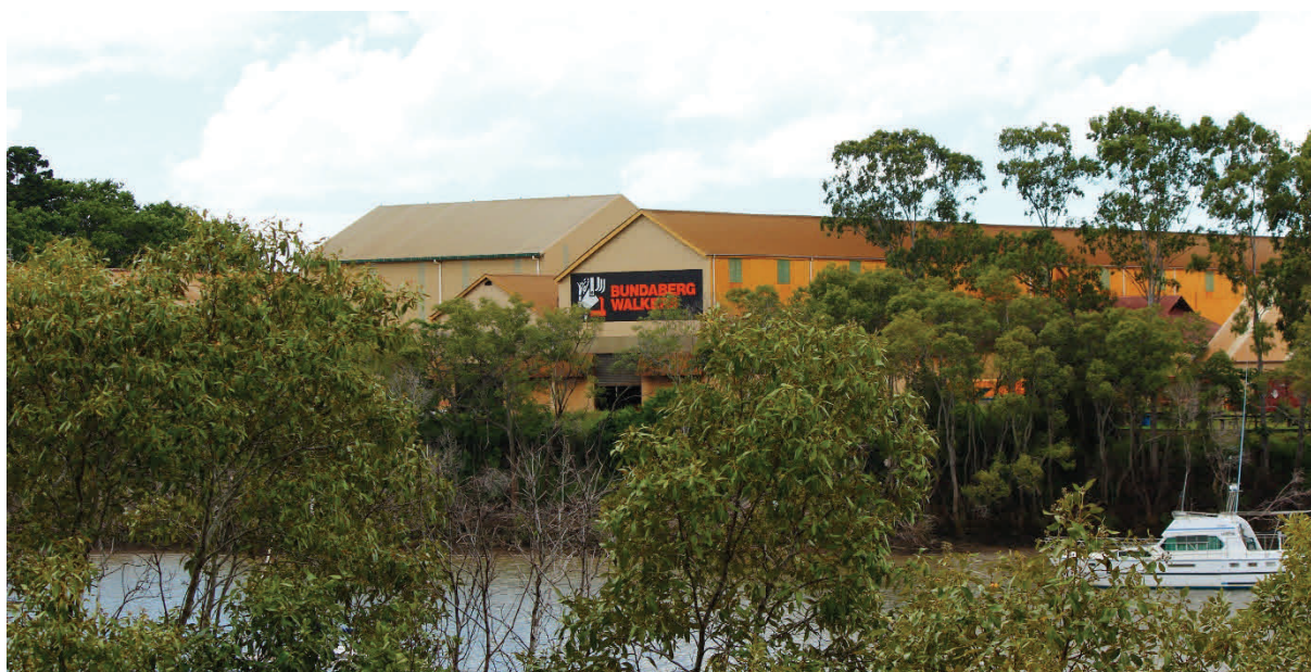
Bundaberg Walkers Engineering Ltd (Foundry), looking across the Burnett River from the south, 3 March 2012. Photo: Kym Browne
