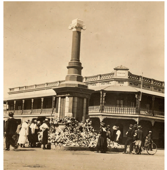
The Metropolitan Hotel stands behind the almost-finished ANZAC memorial statue (the soldier would be placed on top on 7 July 1921), 1921. (bun00286).
