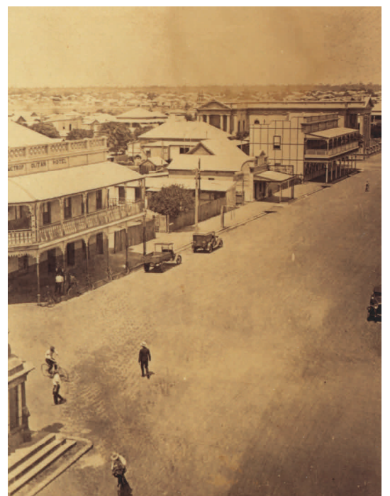
Barolin Street, Bundaberg, with Metropolitan Hotel on left. (bun01608).
